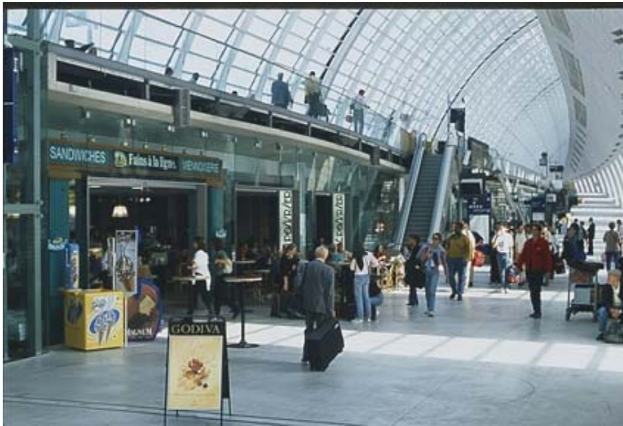
Avignon Railway Station
