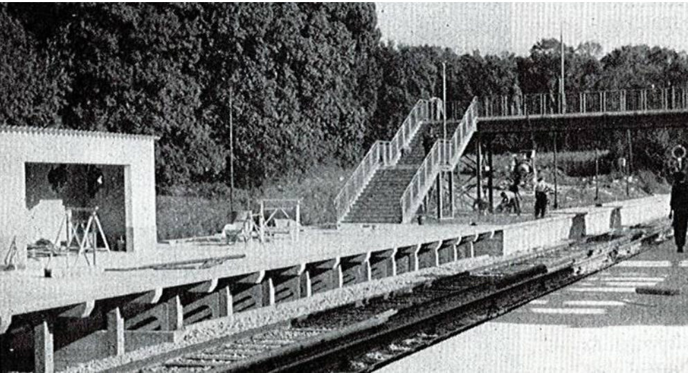
Prefabricated high platforms – La Chataigneraie
