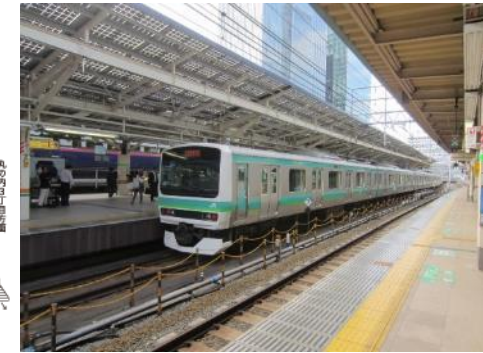
Platform for commuter train
