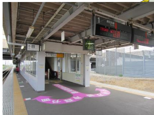
Platform of conventional line
