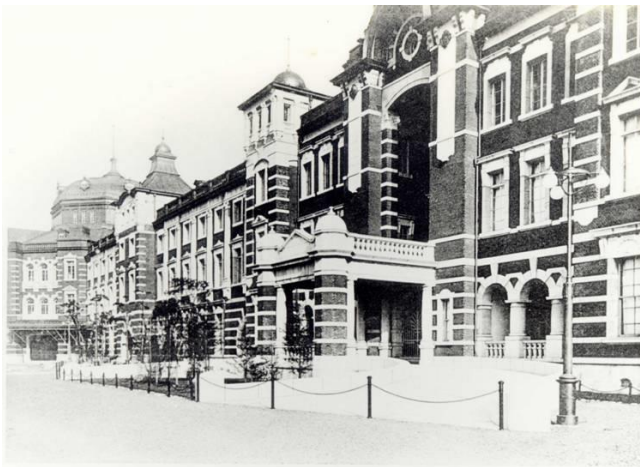
Red brick exterior appearance
