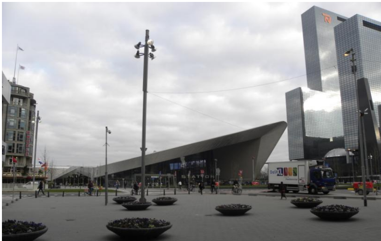
Rotterdam Central Station by Team CS, 2014 © MTriggianese
